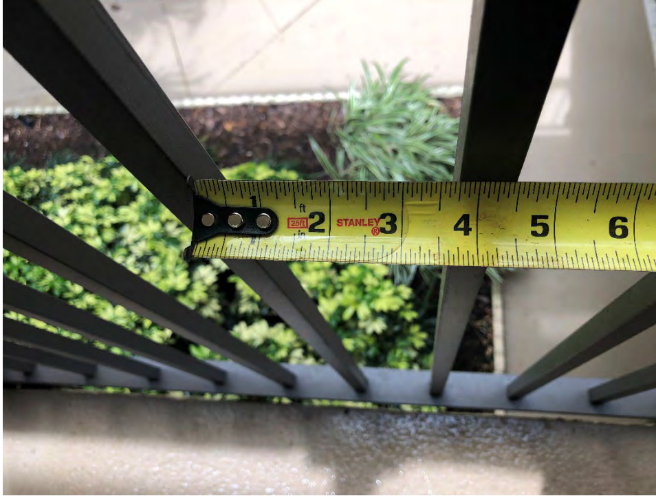
Figure B- 5 – Typical Guardrail Clear Spacing
