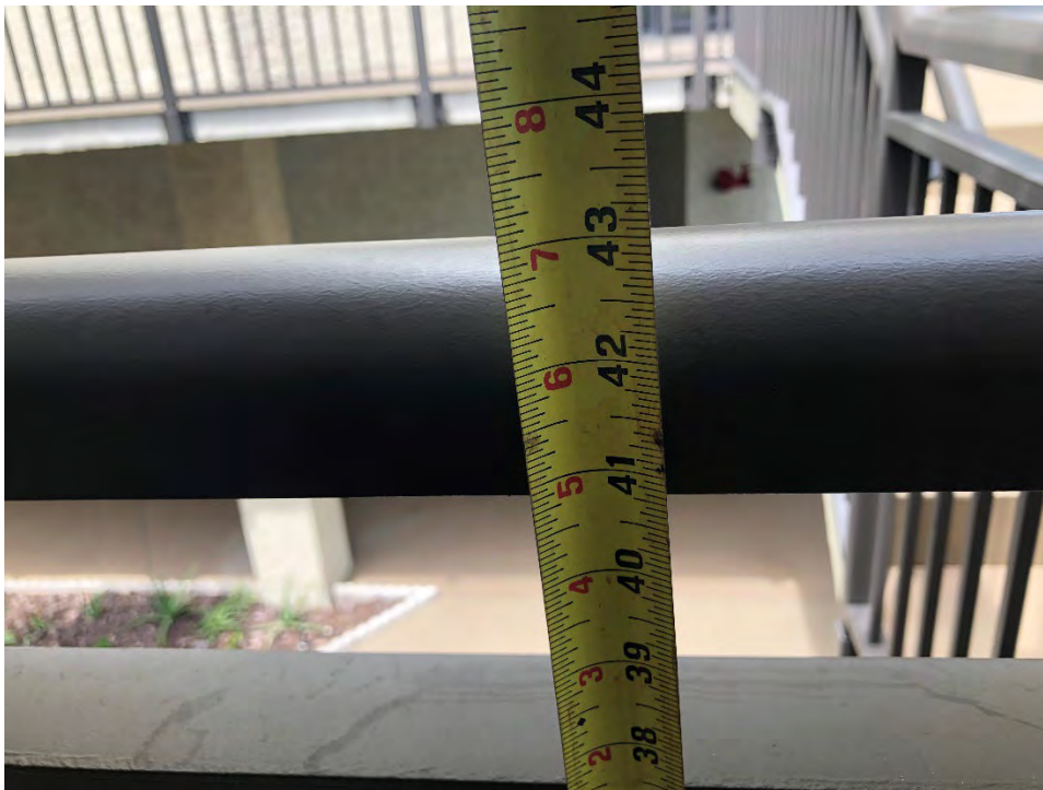
Figure B- 6 – Typical Guardrail Height
