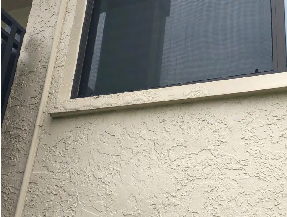
Figure E- 59 – Typical Metal Flashing at Windowsill
