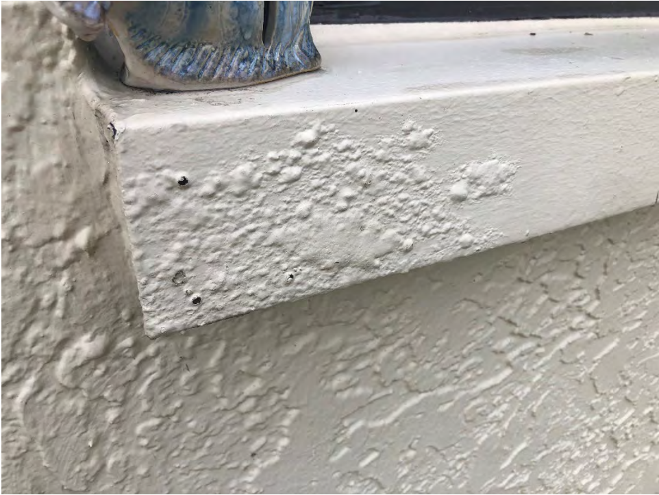
Figure E- 56 – Typical Metal Flashing at Windowsill
