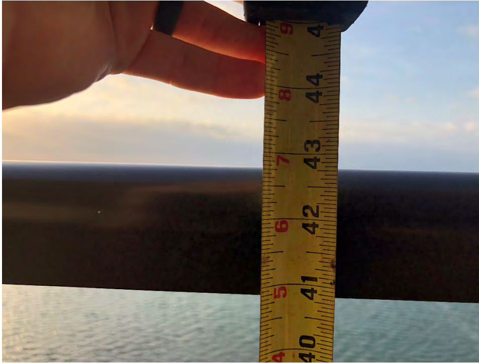
Figure A- 3 – Typical Tower Guardrail Height
