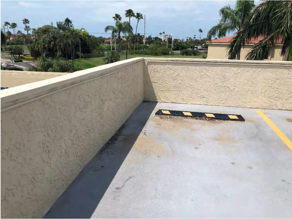
Figure D- 9 – Typical Concrete Guardrail
