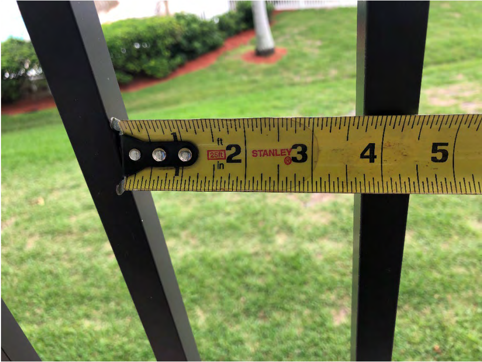
Figure A- 12 – Typical Villa Guardrail Clear Spacing
