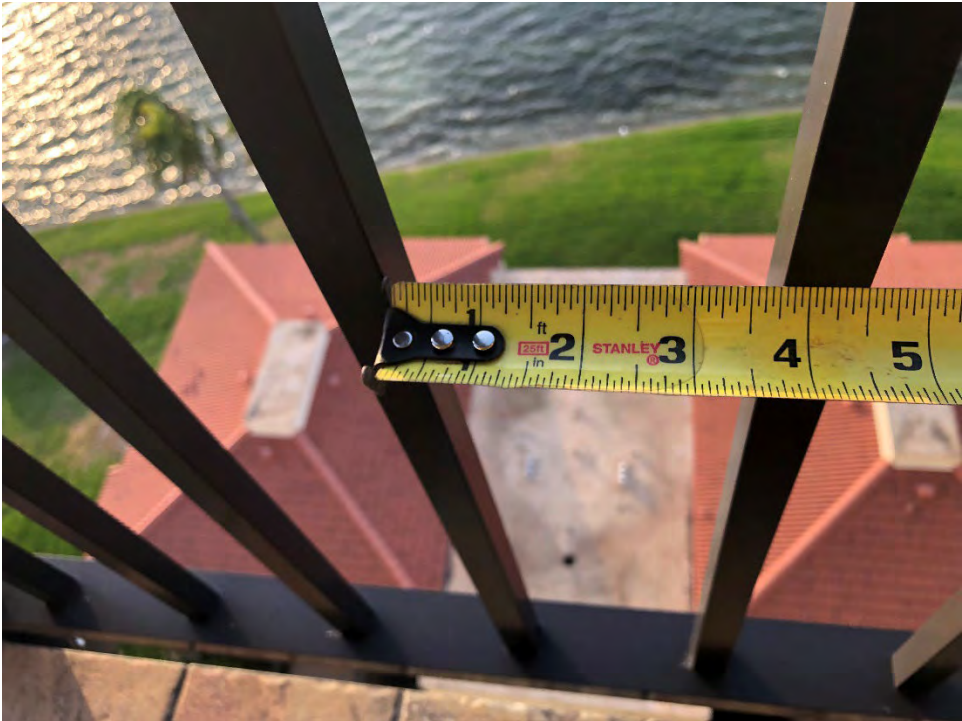
Figure A- 2 – Typical Tower Guardrail Clear Spacing
