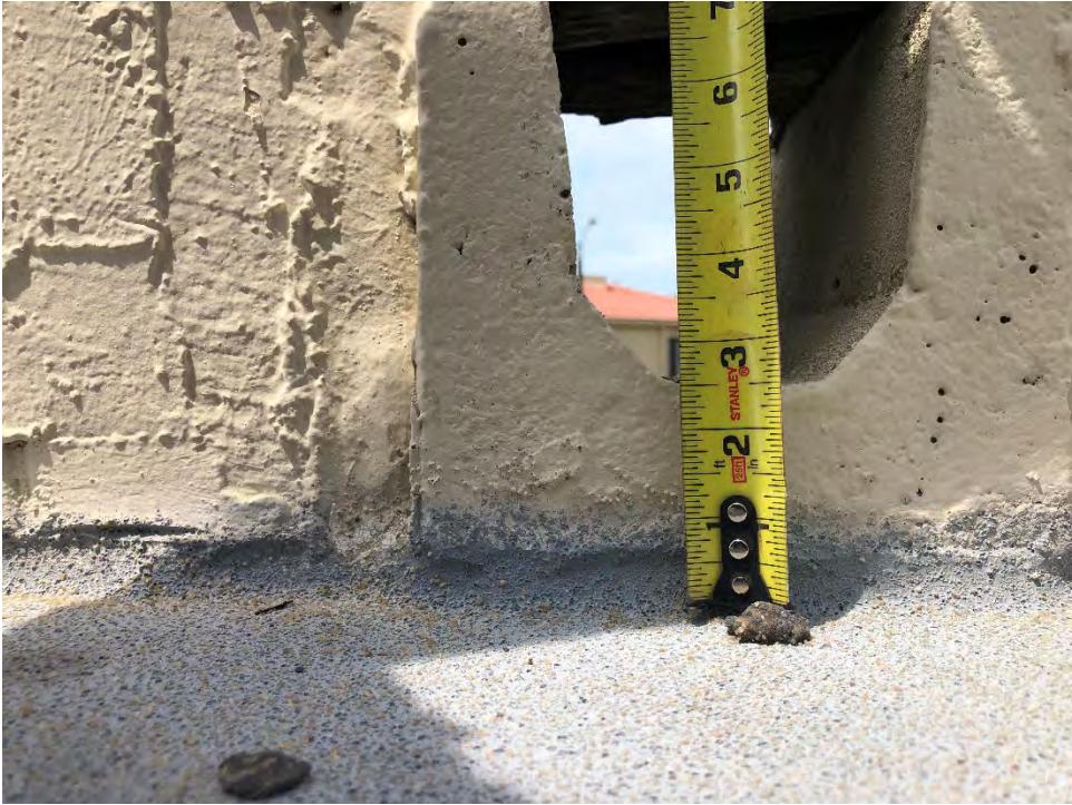
Figure D- 13 – Typical Drainage Scupper
