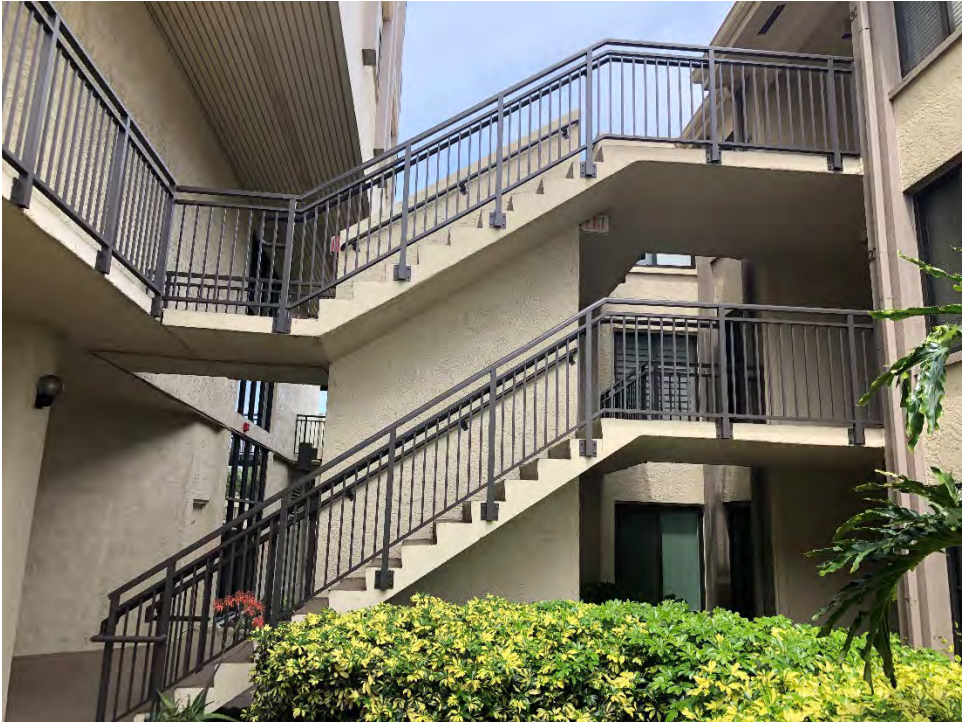
Figure B- 3 – Typical Guardrails
