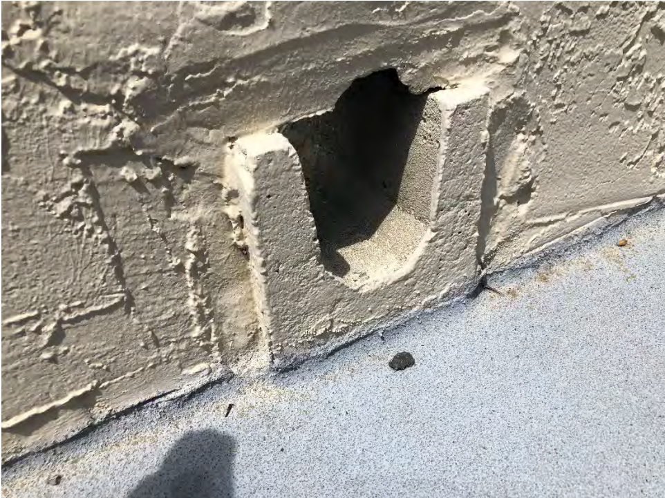
Figure D- 12 – Typical Drainage Scupper
