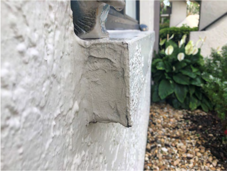
Figure E- 55 – Typical Metal Flashing at Windowsill
