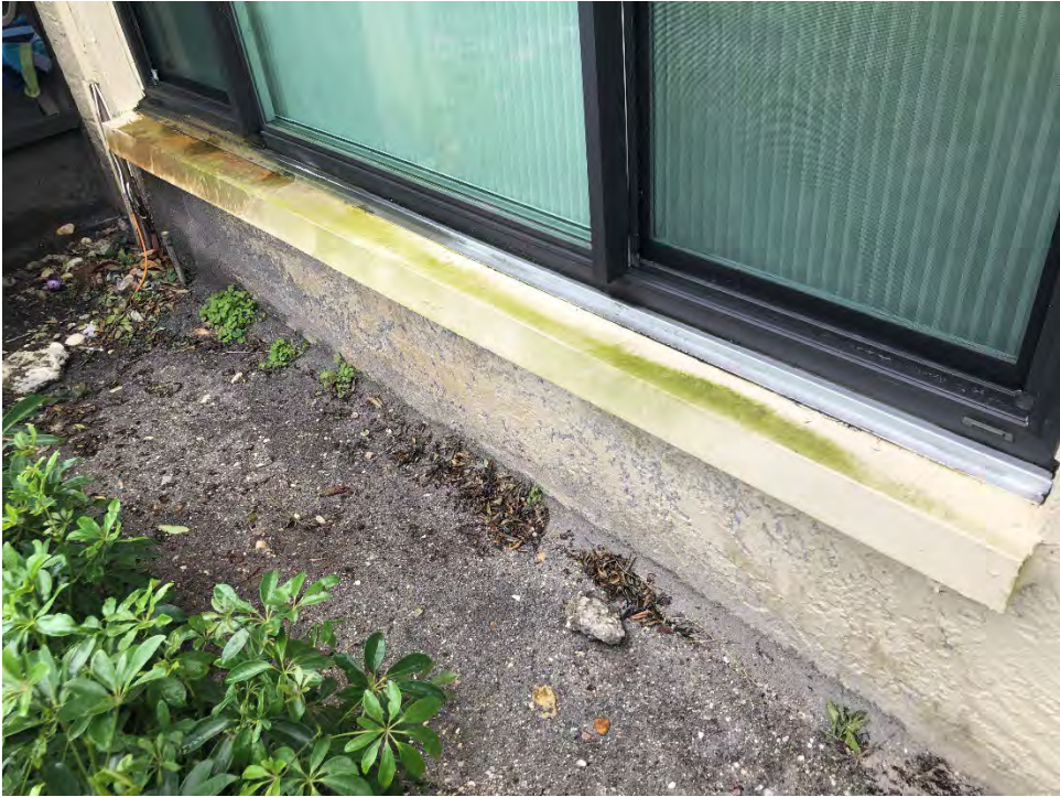
Figure E- 58 – Typical Metal Flashing at Windowsill
