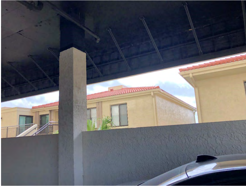
Figure E- 5 – Drop Down Walls/Beams
