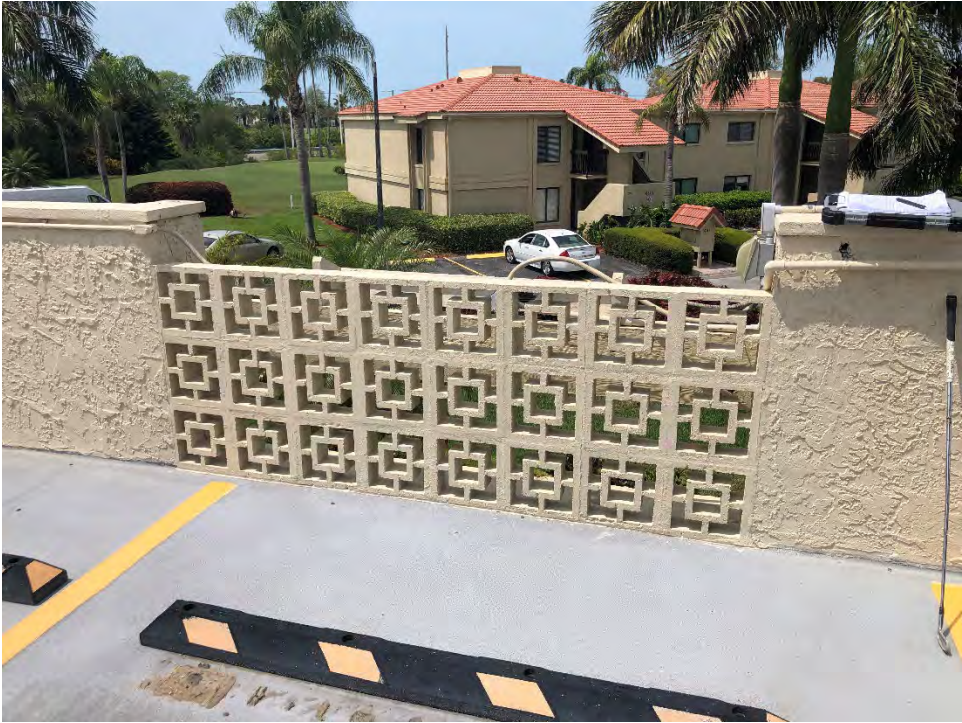
Figure D- 10 – Typical Concrete Guardrail
