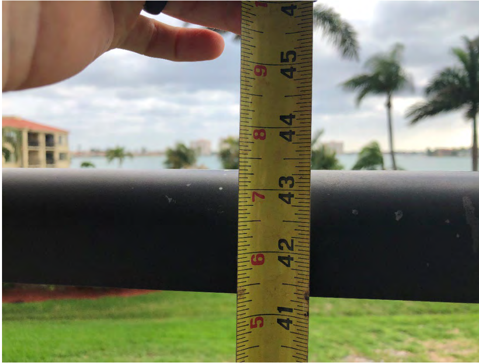
Figure A- 13 – Typical Villa Guardrail Height
