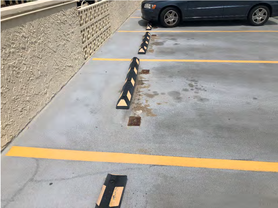
Figure D- 11 – Unadhered Parking Stops
