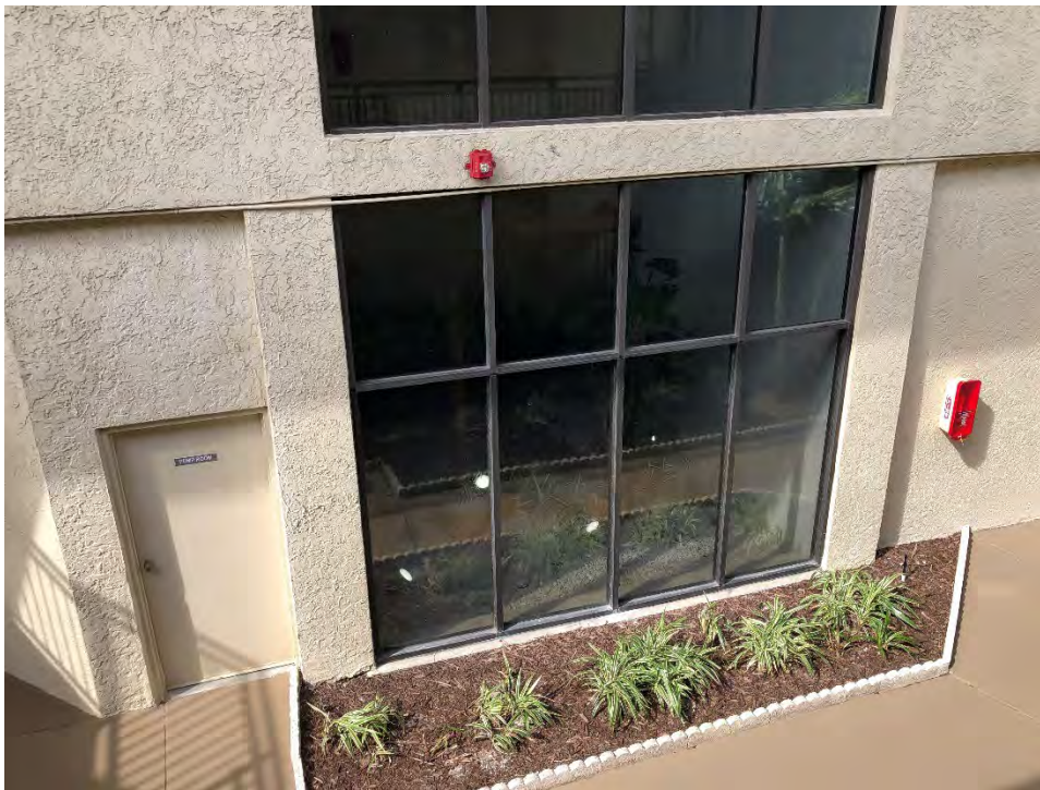
Figure E- 8 – Typical Storefront Windows
