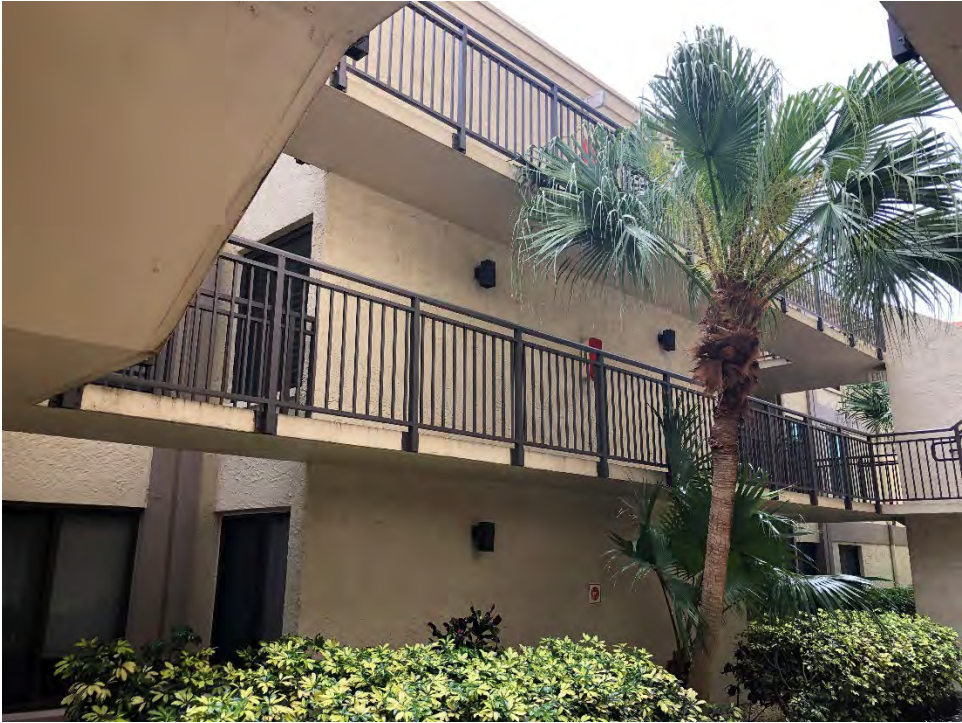
Figure B- 4 – Typical Guardrails
