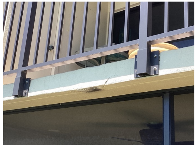
Balconies – railing connection detail
