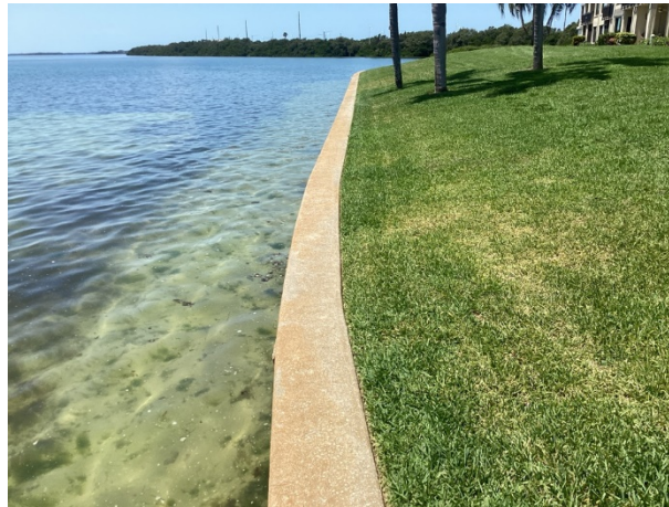
Concrete seawall - overview
