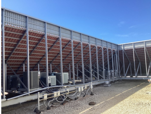
Steel structure - overview
