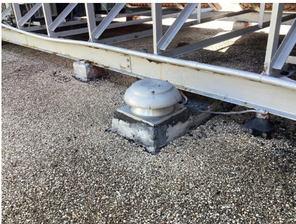
Built-up roof – penetration detail
