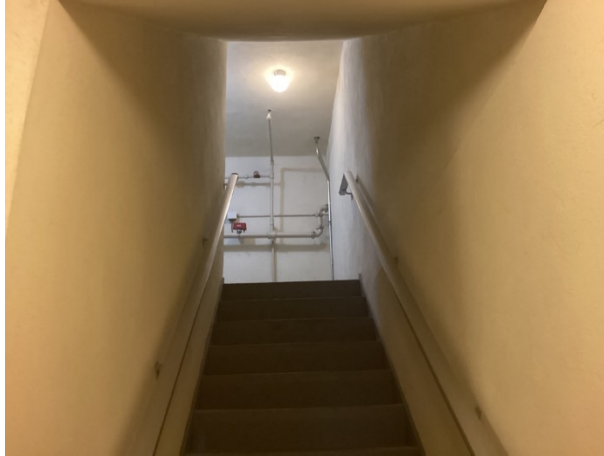
Paint finishes – stairwells - overview
