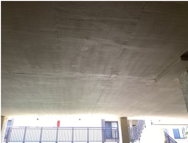
Elevated concrete - overview
