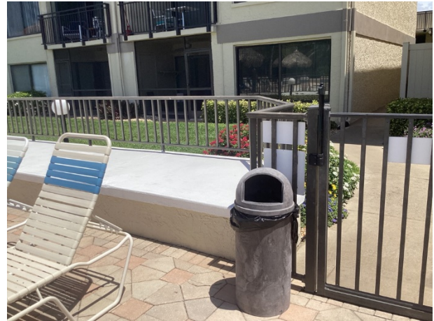
Pool fences - overview
