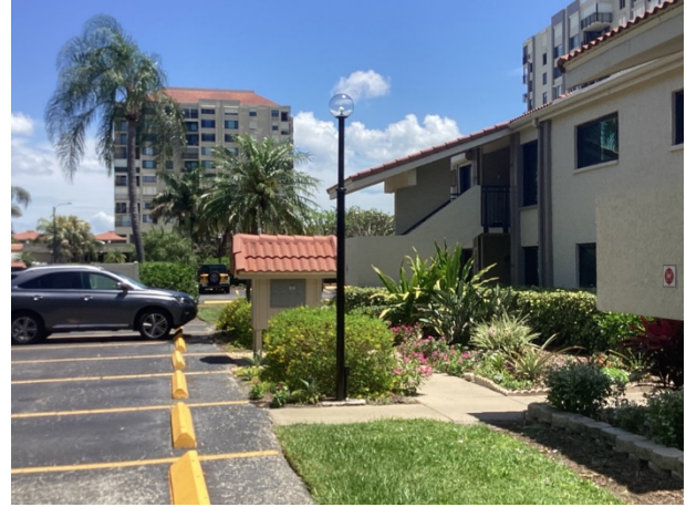
Light pole and fixture
