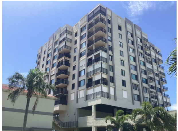
Paint finishes – tower - overview
