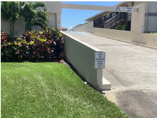
Paint finishes – tower - overview
