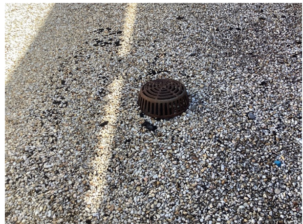
Built-up roof – penetration detail
