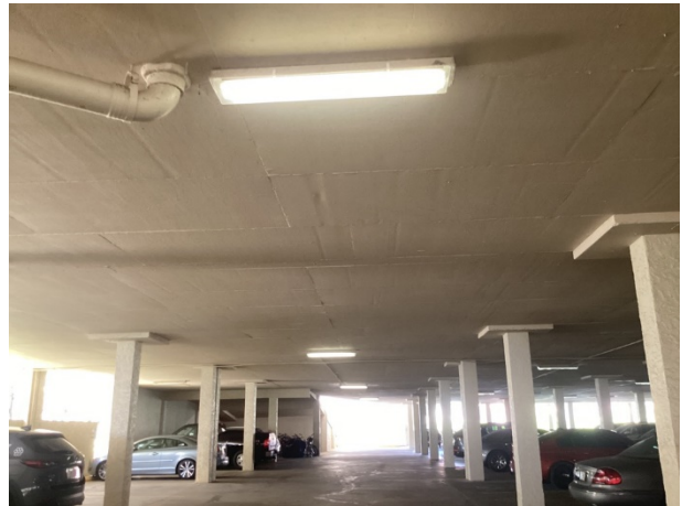
Elevated concrete - overview
