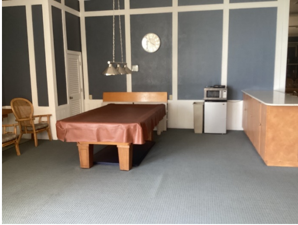
Social room renovation - overview
