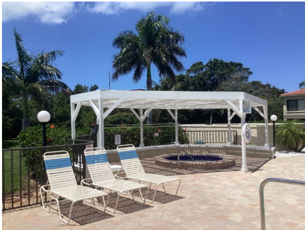
Shade structure - overview
