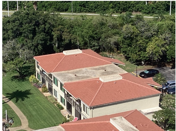
Built-up roof – villa configuration
