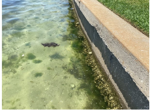
Concrete seawall - overview
