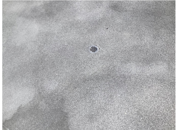
Elevated concrete – drainage detail evident
