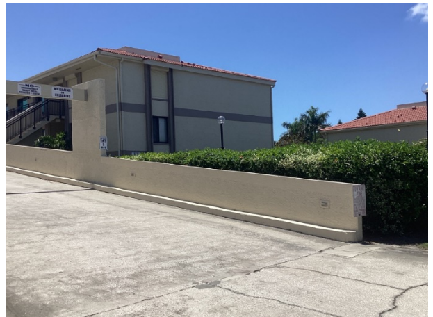
Paint finishes – tower - overview
