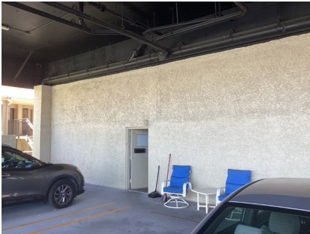
Paint finishes – tower - overview
