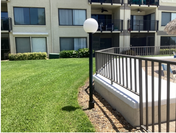
Light pole and fixture
