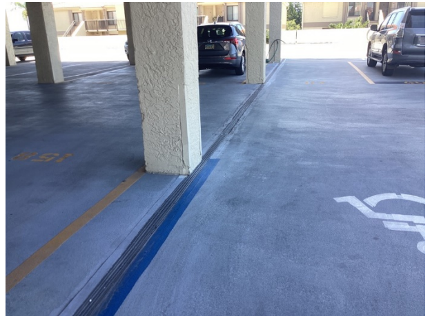
Paint finishes – tower - overview
