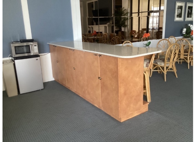
Social room renovation - overview
