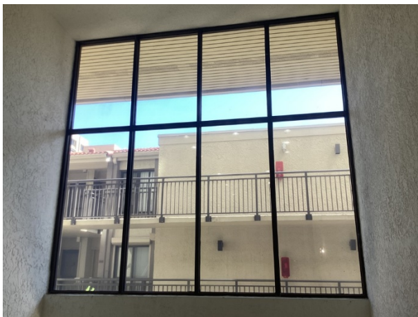
Storefront windows - overview
