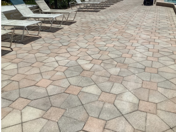
Deck pavers - overview
