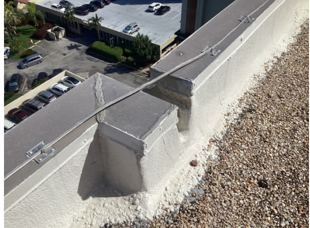
Built-up roof – coping detail
