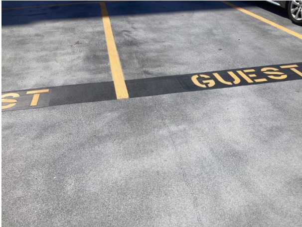
Elevated concrete - overview
