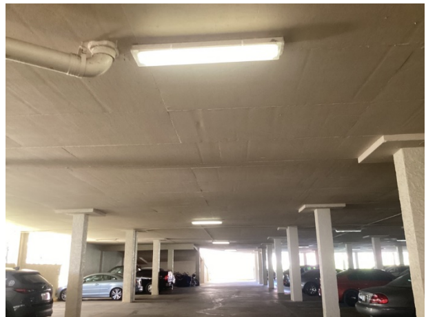
Elevated concrete - overview
