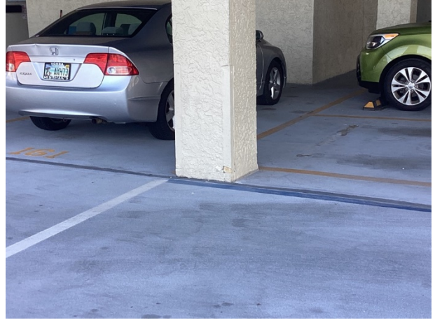
Paint finishes – tower - overview
