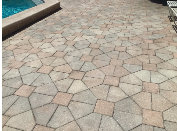
Deck pavers - overview
