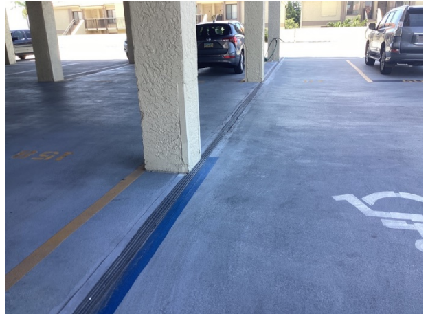
Paint finishes – tower - overview
