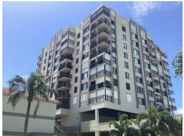
Paint finishes – tower - overview
