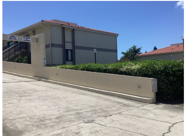
Paint finishes – tower - overview
