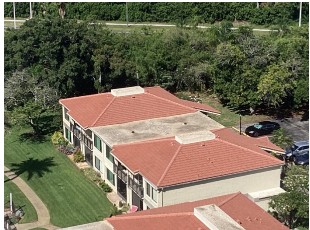
Built-up roof – villa configuration
