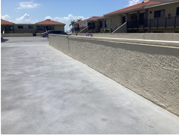
Paint finishes – tower - overview
