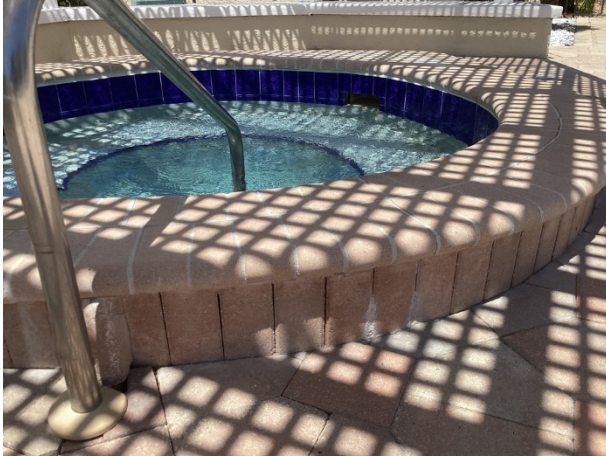
Spa finishes - overview
