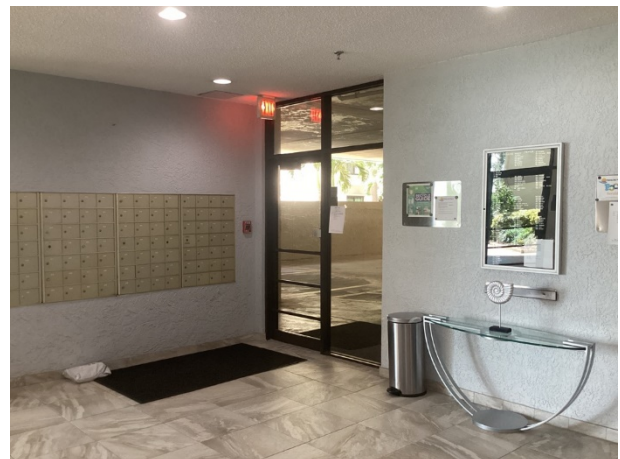
Storefront windows and doors – overview
