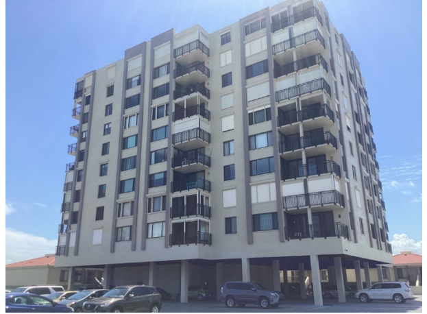
Paint finishes – tower - overview
