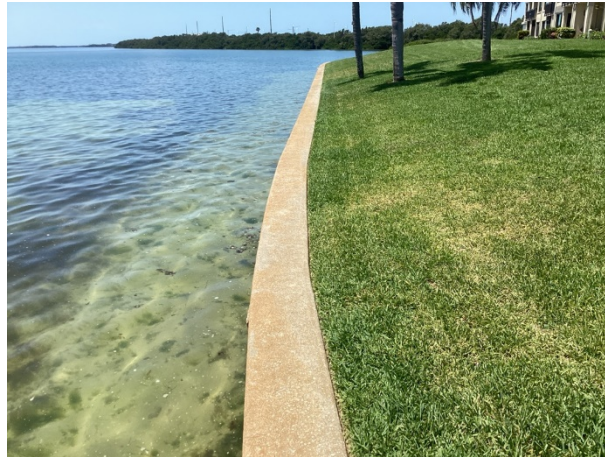
Concrete seawall - overview
