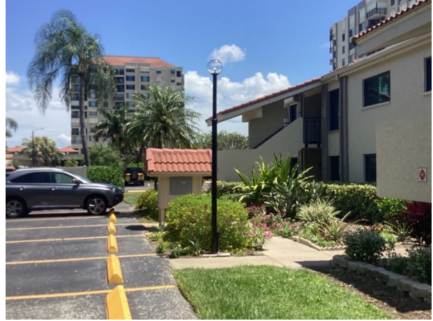
Light pole and fixture
