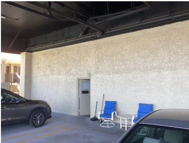
Paint finishes – tower - overview
