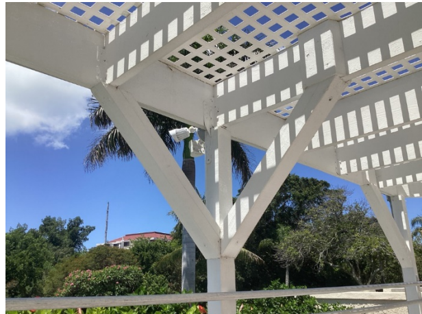
Shade structure – support detail
