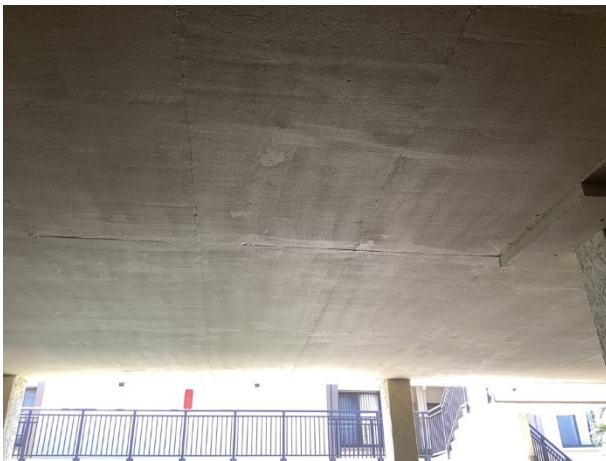
Elevated concrete - overview
