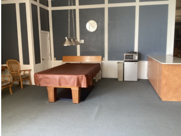
Social room renovation - overview
