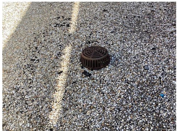
Built-up roof – penetration detail
