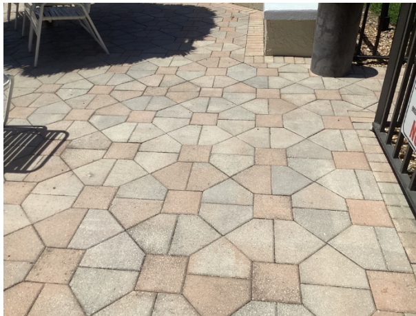
Deck pavers - overview
