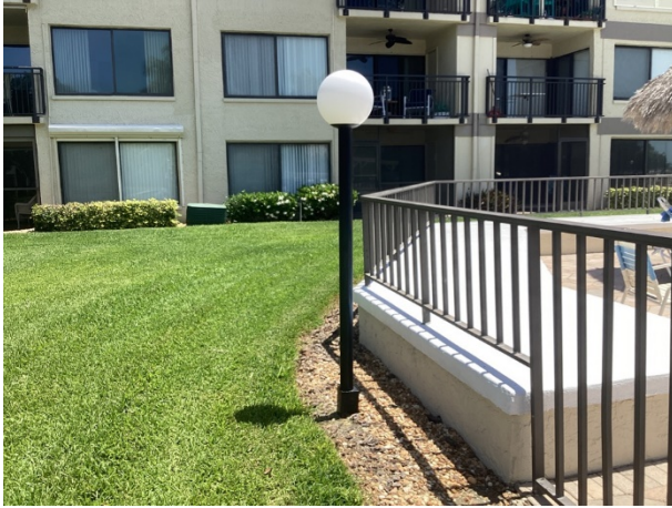
Light pole and fixture
