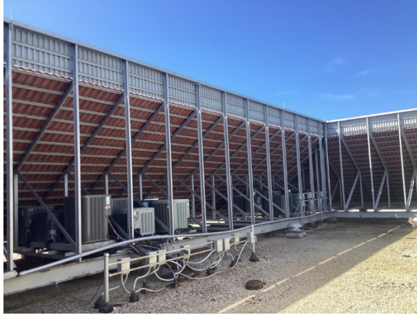
Steel structure - overview
