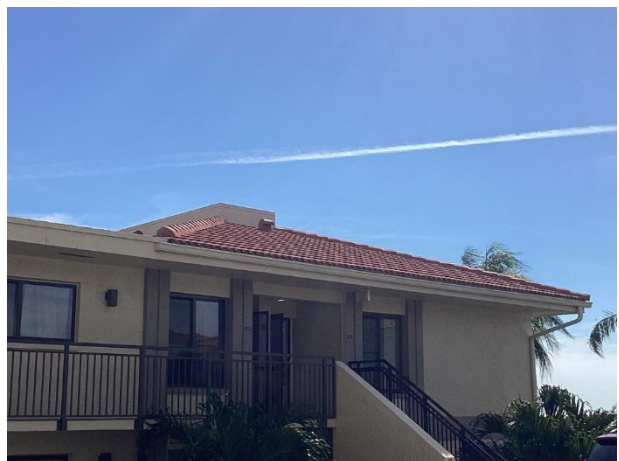
Concrete tile roofs - overview
