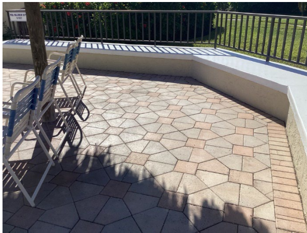
Deck pavers - overview
