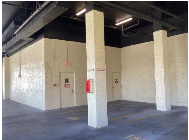
Paint finish applications – Garage - overview
