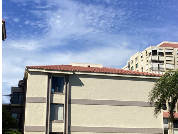
Concrete tile roofs - overview
