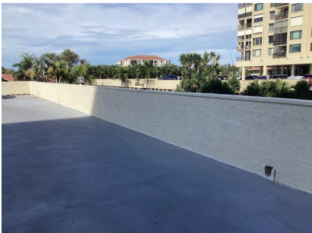
Paint finish applications – Garage - overview
