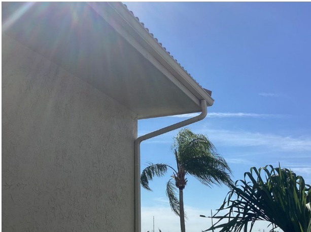
Gutters and downspouts - overview
