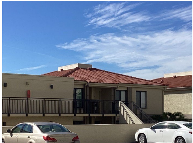
Concrete tile roofs - overview
