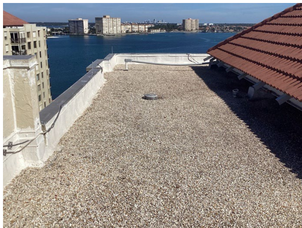
Built-up roof - overview
