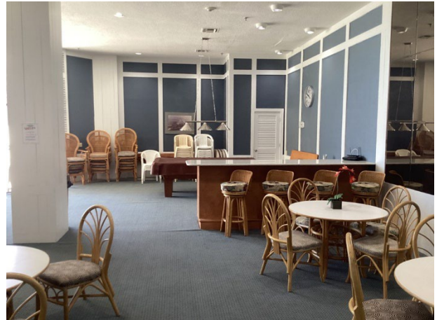
Social room renovations - overview
