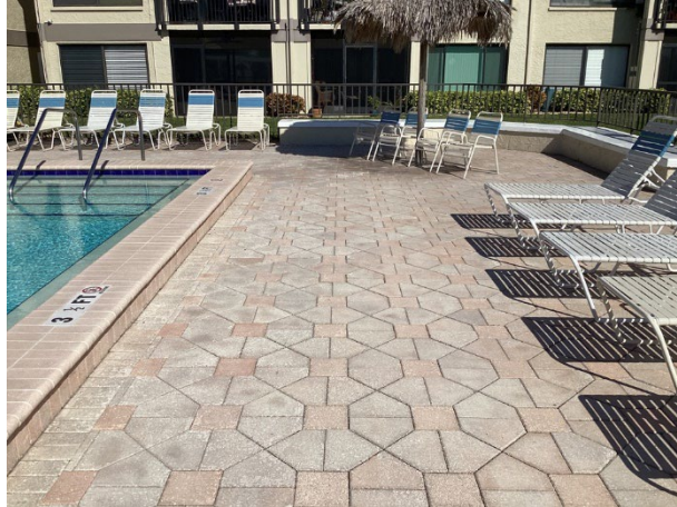
Deck pavers - overview
