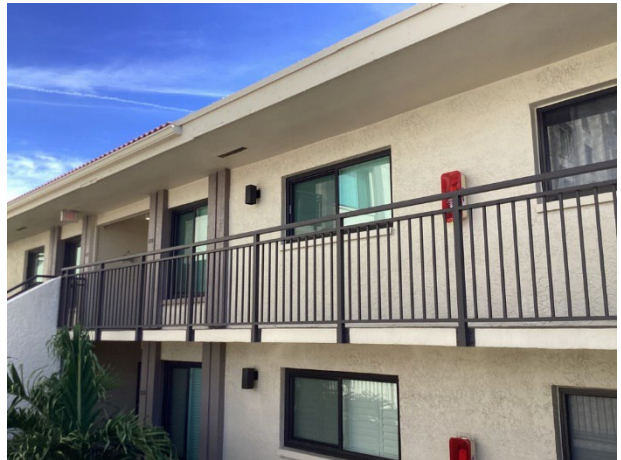
Paint finish applications – Villas - overview
