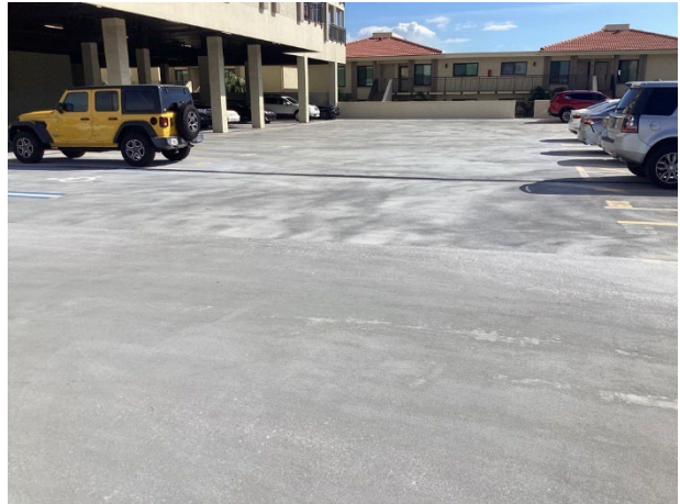
Elevated concrete - overview
