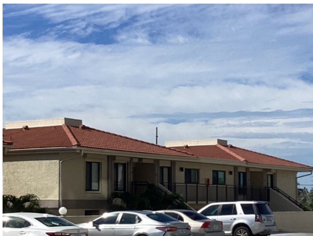
Concrete tile roofs - overview
