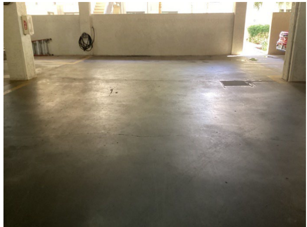
On-grade concrete – overview
