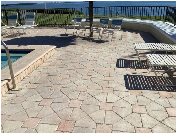
Deck pavers - overview
