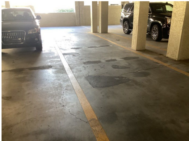
On-grade concrete – overview
