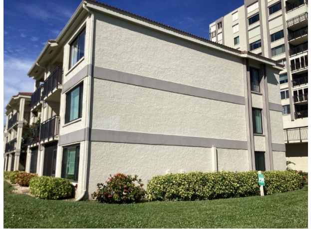
Paint finish applications – Villas - overview
