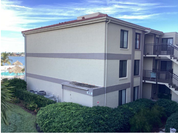
Paint finish applications – Villas - overview
