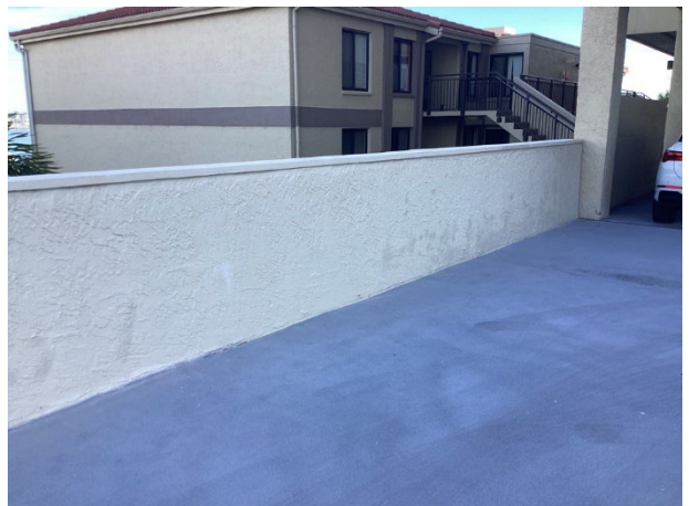
Paint finish applications – Garage - overview
