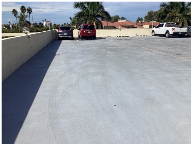
Elevated concrete - overview
