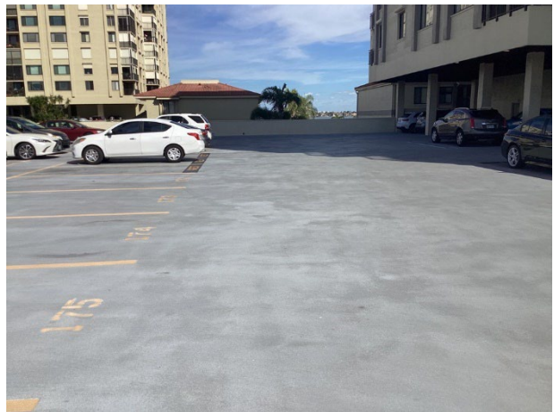
Elevated concrete - overview
