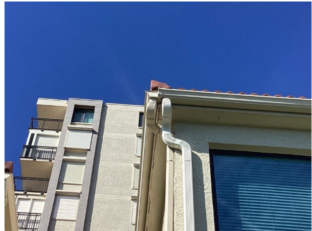
Gutters and downspouts - overview
