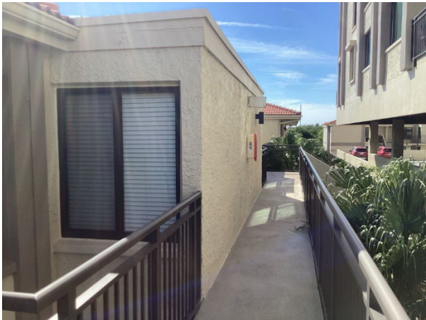
Paint finish applications – Villas - overview
