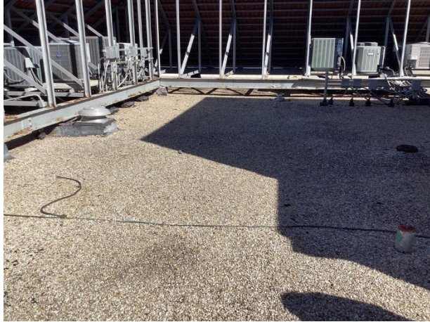
Built-up roof - overview
