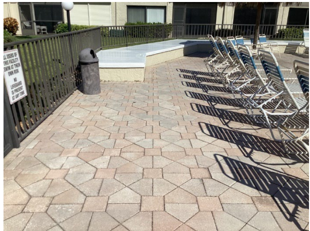
Deck pavers - overview
