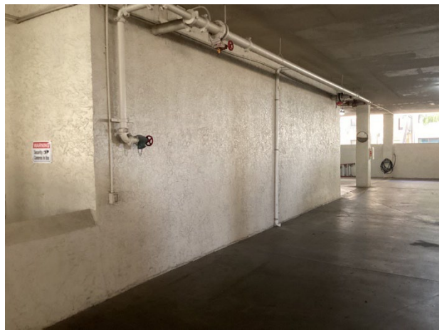
Paint finish applications – Garage – overview
