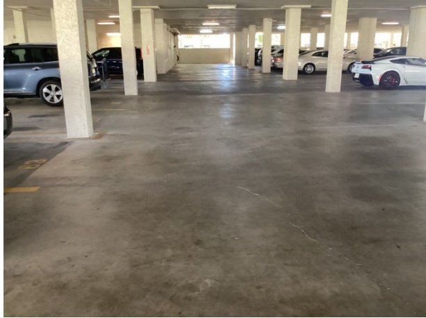
On-grade concrete – overview
