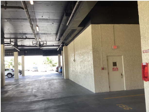
Paint finish applications – Garage - overview
