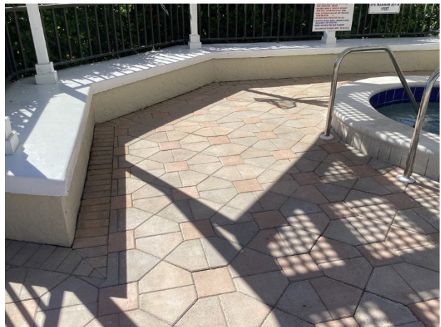
Deck pavers - overview
