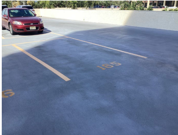
Elevated concrete - overview
