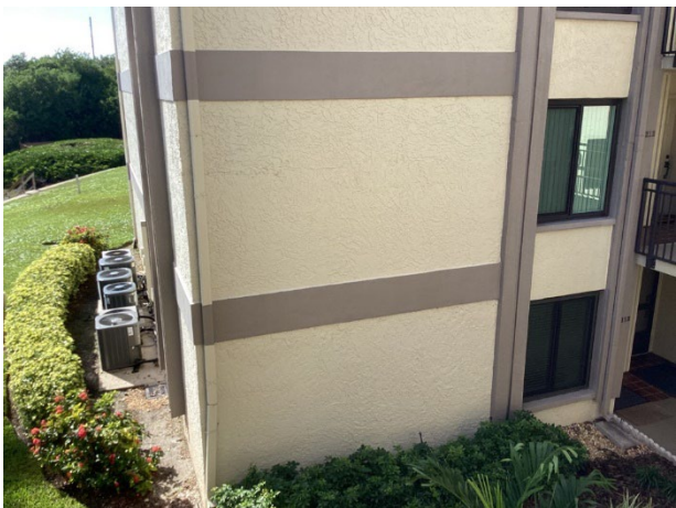
Paint finish applications – Villas - overview
