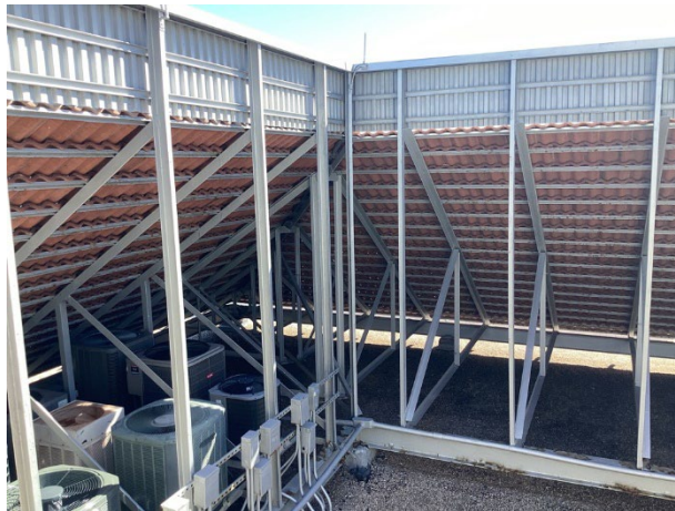
Steel structure – overview
