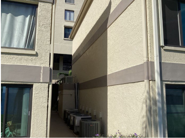
Paint finish applications – Villas - overview
