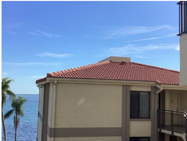
Concrete tile roofs - overview
